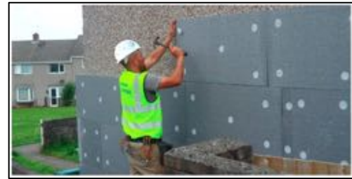
Installing external insulation on a solid wall
