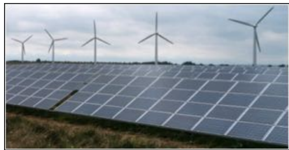
Westmill wind and solar co-op, Watchfield, Oxon
